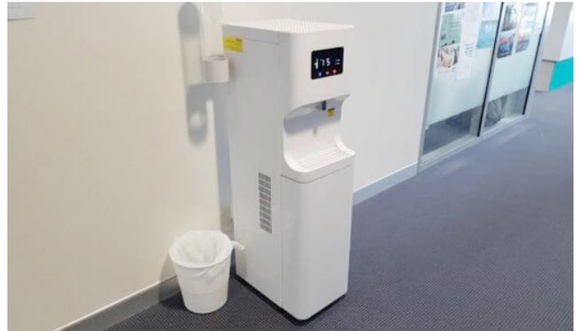
Using state of the art micro pumps, the water is then pumped through the remaining filters, including a sediment filter that eliminates particles over 5 micron in diameter, a pre carbon filter containing activated carbon and coconut shell, an ultra fine membrane filter that eliminates particles as small as 0.01 microns in diameter, followed by a post carbon filter.
